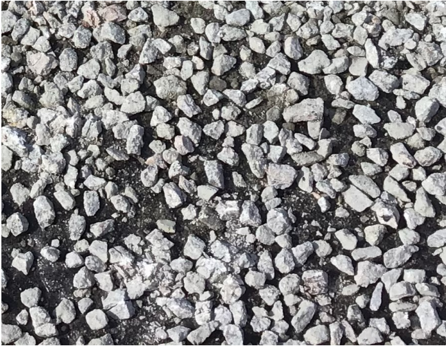
Pictured Above: Mat Seal (HMA Interlayer)
